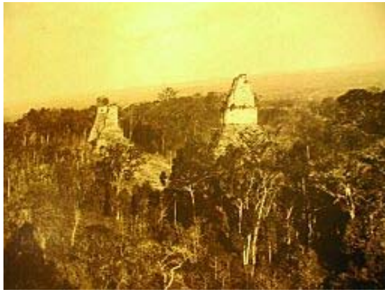
A photo of showing the start of excavation work in the park, compared with a recent photo.
